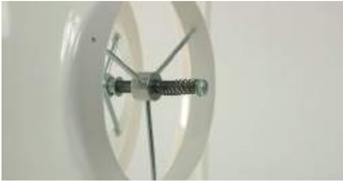
INSTALLATION WITH CONNECTING SLEEVE AND BUTTERFLY DAMPER
